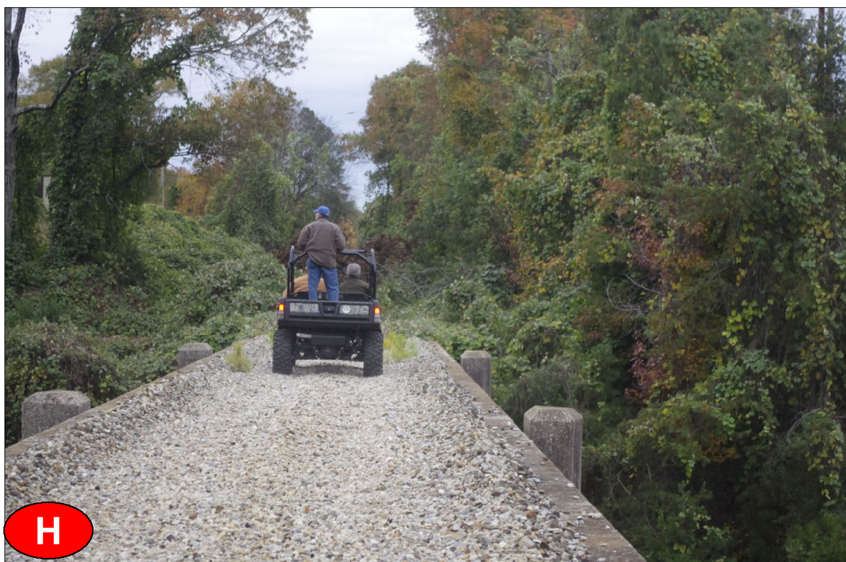
Bridge Over Old US Highway 431
