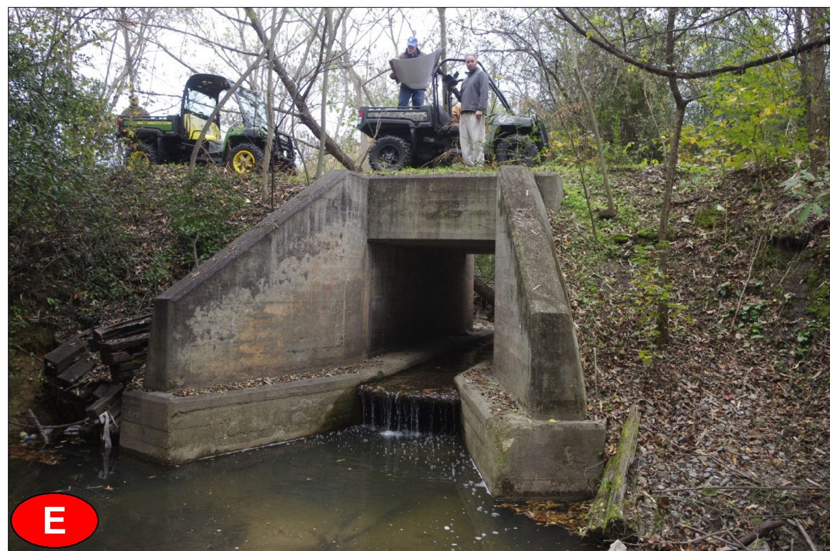
Stream Culvert Near Norwood Park
