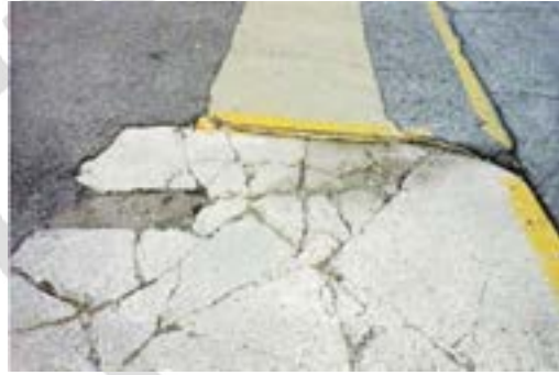
Non-compliant cracks
